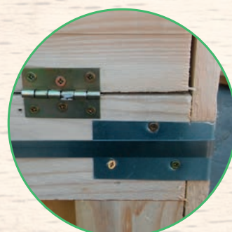
Detail of the connecting material
